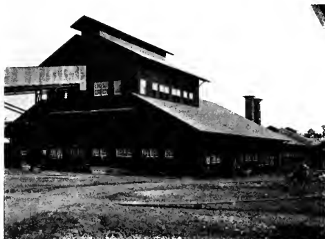
First paper mill in the Hawaiian Islands.—View of the paper mill buildings of the Olaa Sugar Company.
